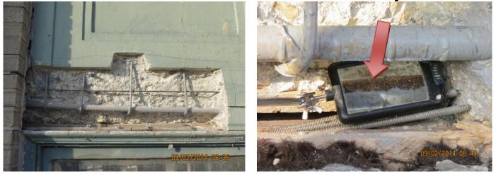
Existing steel which needed to be cleaned and coated was not properly cleaned (wire-wheeled) and coated on the underside...
